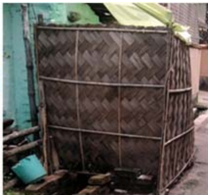
FIGURE 18. a wall of a KUTCHA house made up of bamboo sheets
