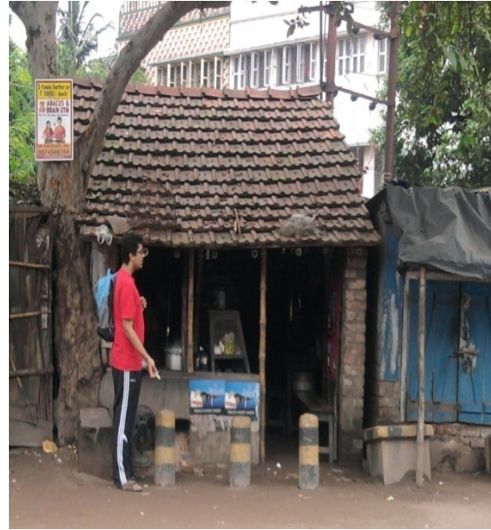
FIGURE 16. A roof made up of mud tiles and unburnt bricks
