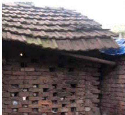
FIGURE 17. KUTCHA house's wall made up of unburnt brick
